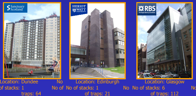
Figure 4: Three buildings used to validate the reflected wave technique during extensive field trials
